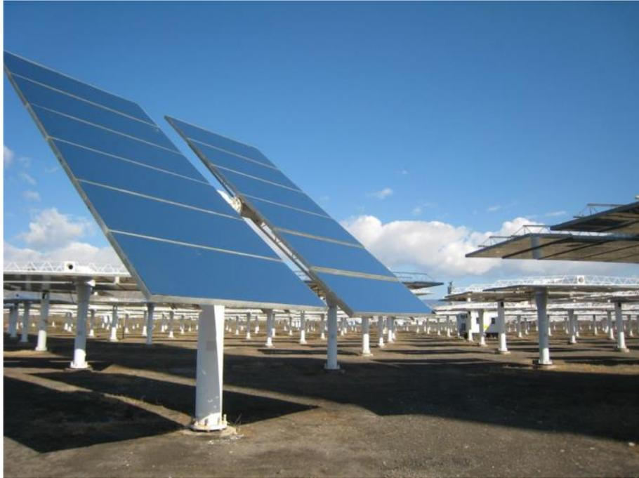
Figure 3.16. New mirror facets installed on the CESA-I heliostat field
