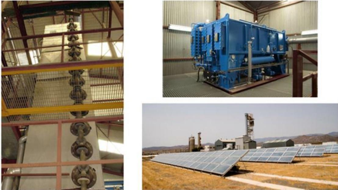
Figure 2.33. The PSA SOL-14 MED Plant (left), double-effect LiBr-H<sub>2</sub>O absorption heat pump (upper right) and 500-m<sup>2</sup> CPC solar collector field (bottom right)
