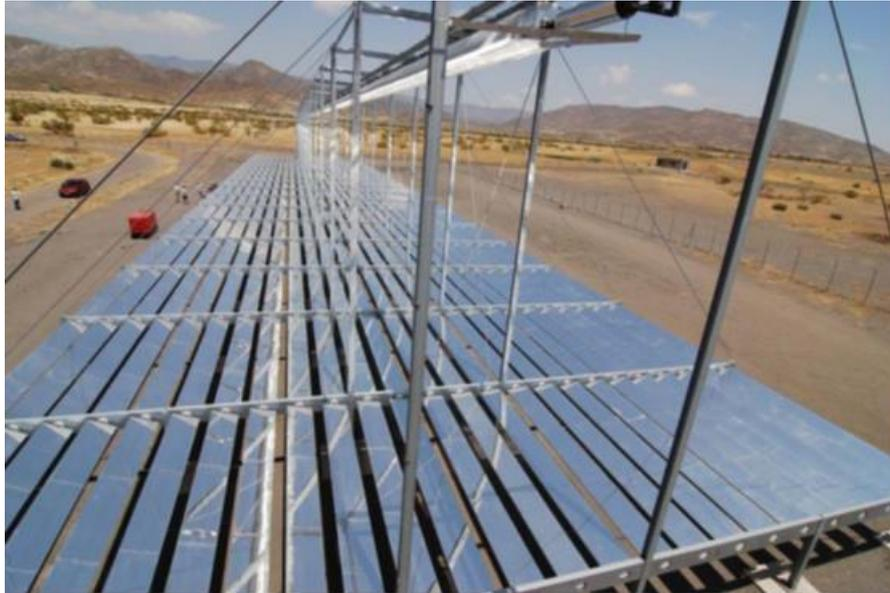
Figure 2.12. Photo of the linear Fresnel concentrator erected at the PSA.
