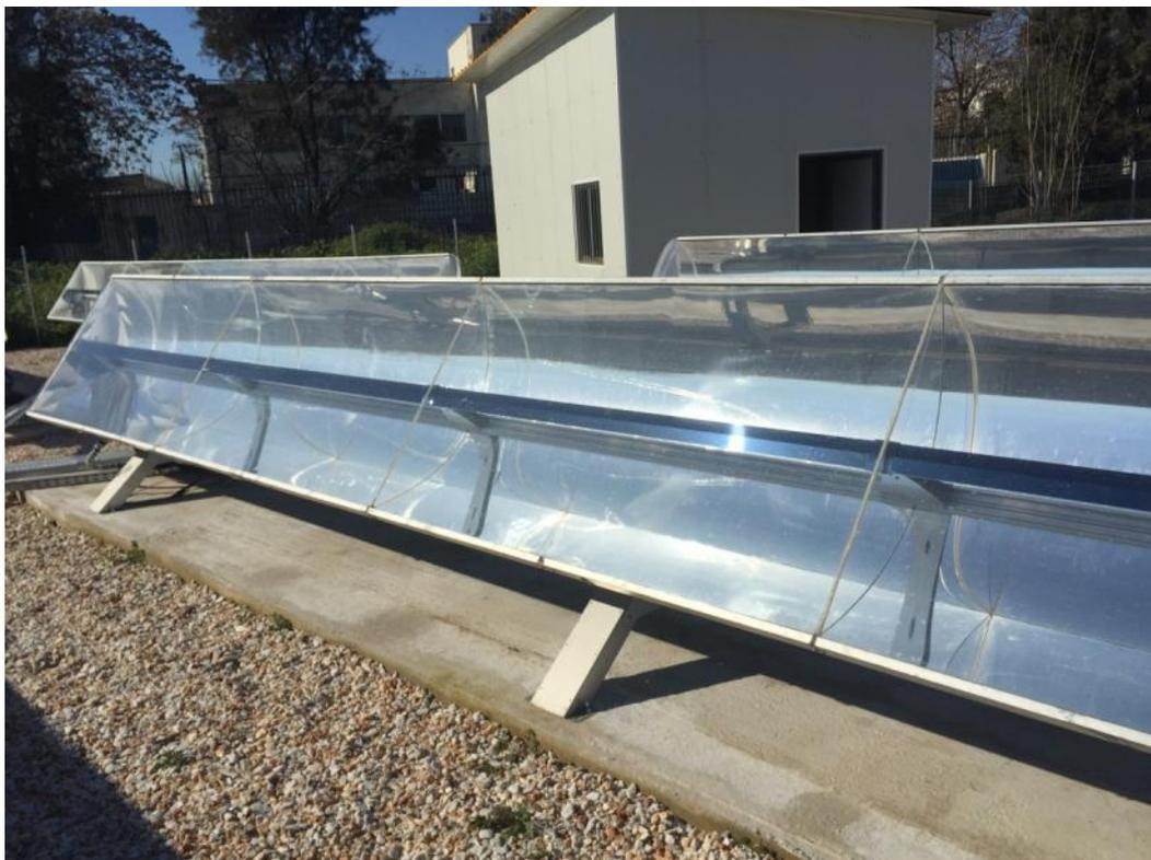
Figure 4.5: Absolicon CPV/T collectors in CPV/Rankine pilot plant
